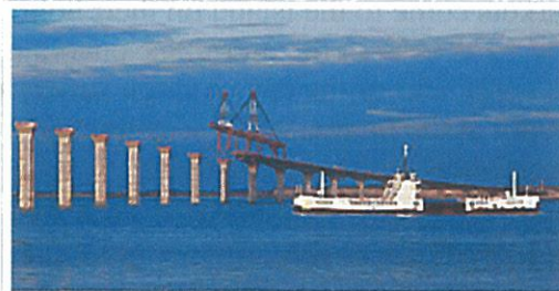
A bac and the bridge under construction, in 1987.
